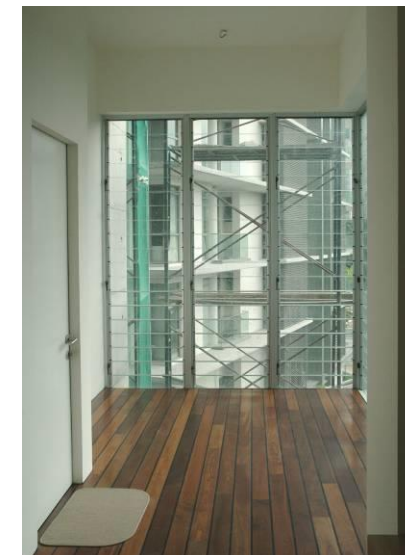
Louvre as partitions with different louvre blade Natural Anodized louvre with aluminium blade, operable via actuators
