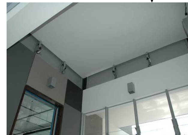
Louvre as partitions with different louvre blade Natural Anodized louvre with aluminium blade, operable via actuators
