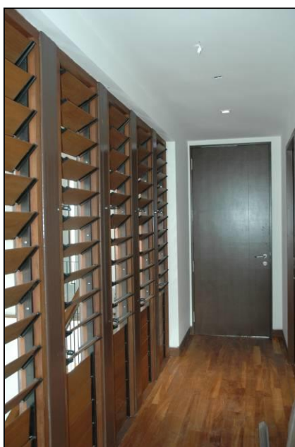
Louvres with timber blades installed along master bedroom's passageway.
